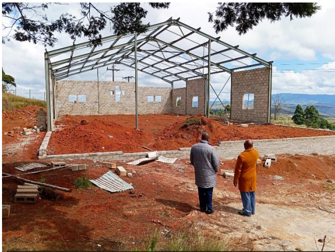
The new Lamb of God Building under construction.
